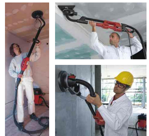
Can sand 3m high ceilings & wall surfaces
